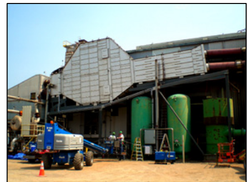
ENDURE™ SCR system for 13 megawatt application
